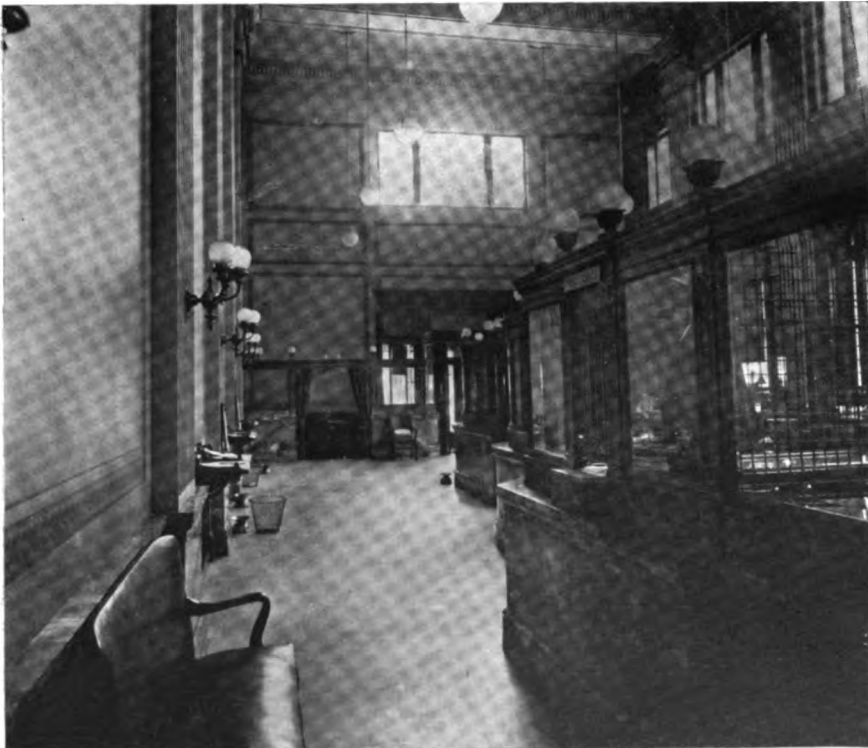
Looking Down the Public Lobby Towards the Main Entrance.
